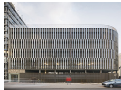
Danube vert - parking silo, Strasbourg (67)
